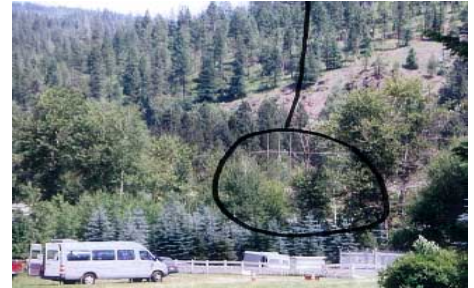
Photo: Barbara Miller. Utility wires located 40 feet in height that may get raised to 60 feet because of a toxic waste dump in northern Idaho.
